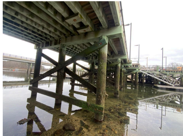
Piles, Bracing, and Pile Caps
