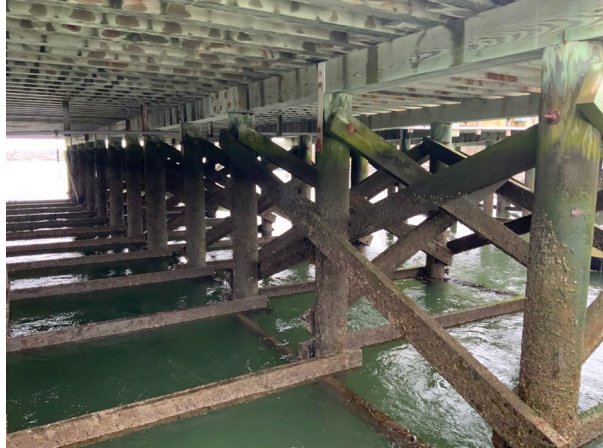
Piles, Bracing, and Pile Caps
