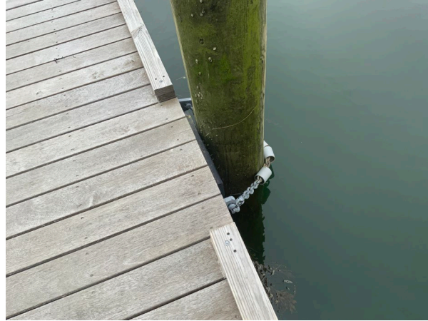
Guide Piles and Assemblies
