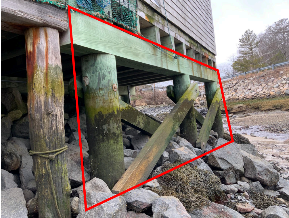
Piles, Bracing, and Pile Caps
