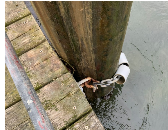
Guide Pile Assembly
