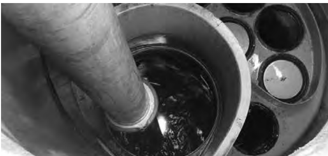
Vacuuming Sump Through MAW
