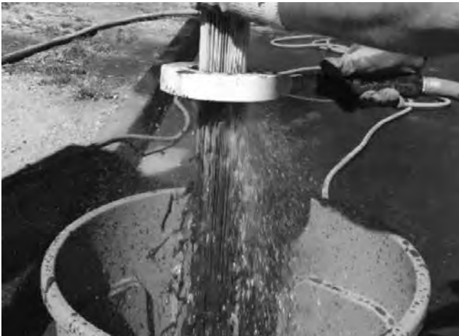
Rinsing Cartridge with Contech Rinse Tool
