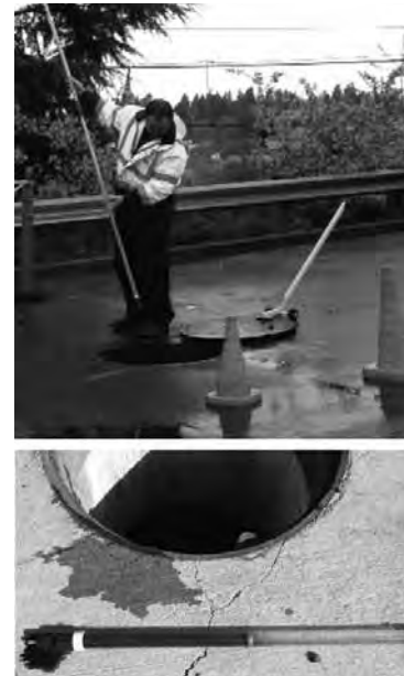
Inspection Utilizing Sediment Probe
